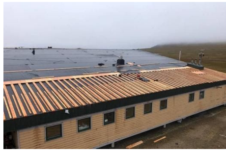
New roofing being installed
