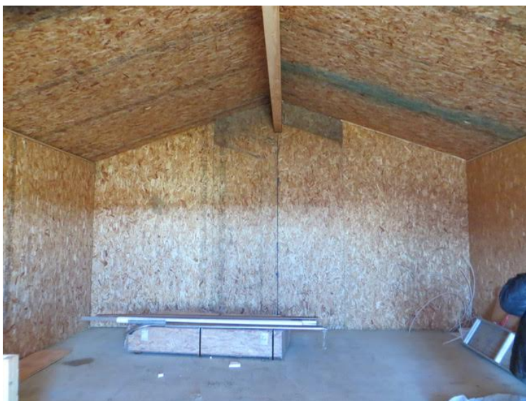
Elim school vehicle garage under construction.
