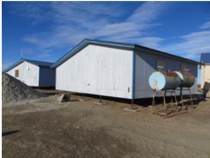
2 Shishmaref portable classrooms at their new location waiting to be converted into teacher-housing duplexes.
