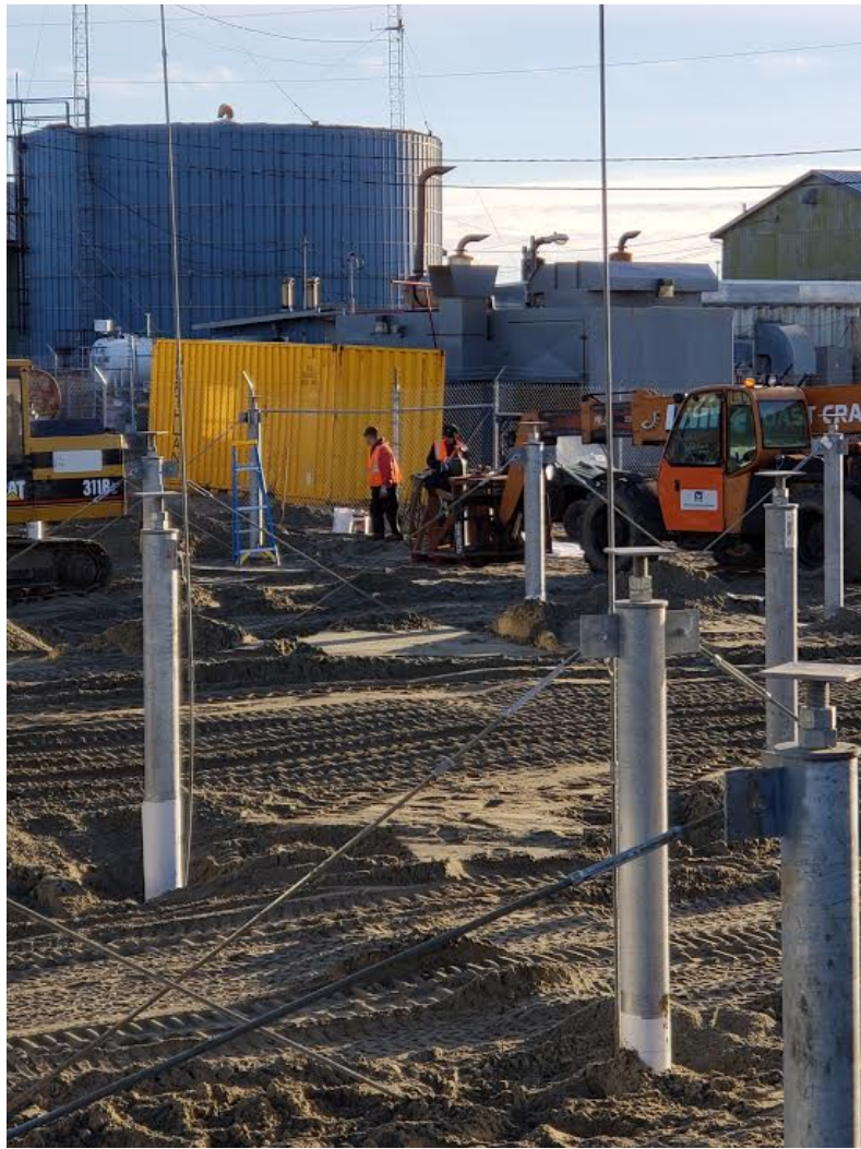
Shishmaref. Building foundation work taking place for the new Elem addition.
