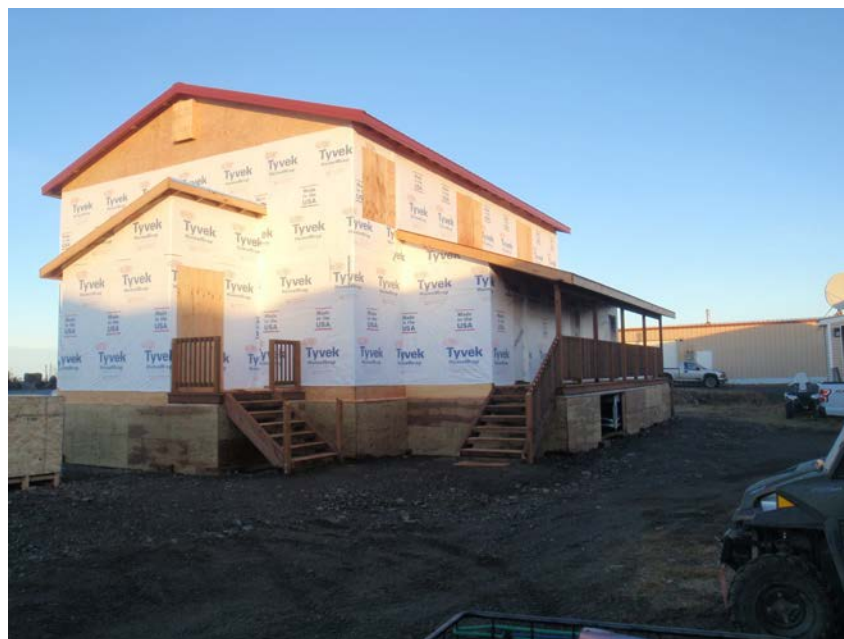
Unalakleet tri-plex under construction.
